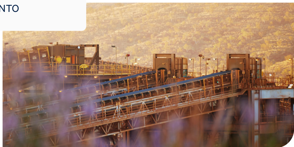
Solomon Mine Ore Processing Facility
