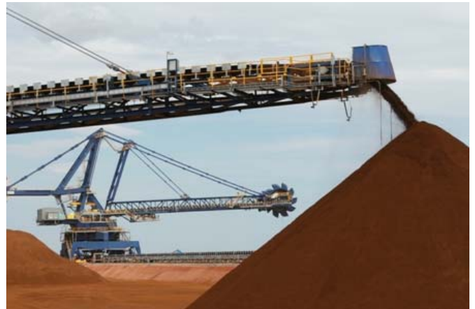
Stacker & Reclaimer Port Site
