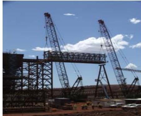
*CV106 Shuttle Truss at Screenhouse*
