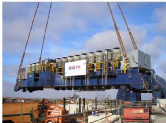
**Ore Car Indexer being lowered into position**
