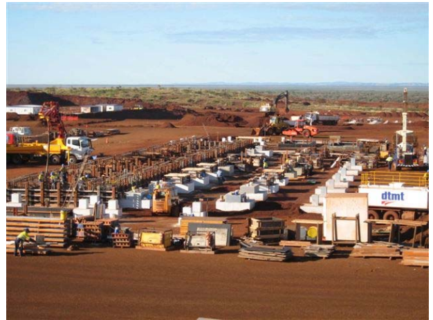
Screening building foundations
